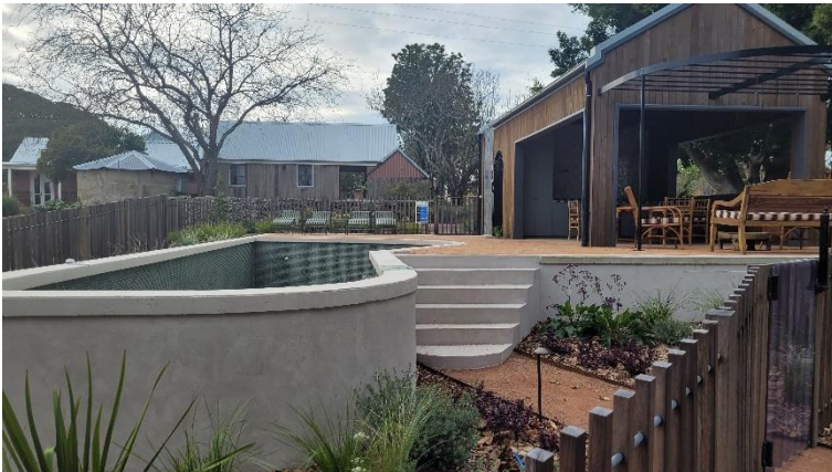
Photo 39 View of new commercial and recreational structures and landscaped gardens in the Greyleigh homestead complex
