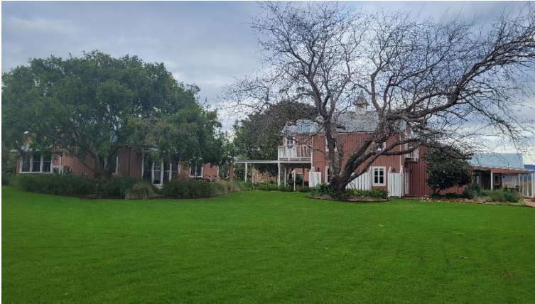
Photo 38 View of the Greyleigh homestead complex showing residential or commercial buildings and landscaped gardens
